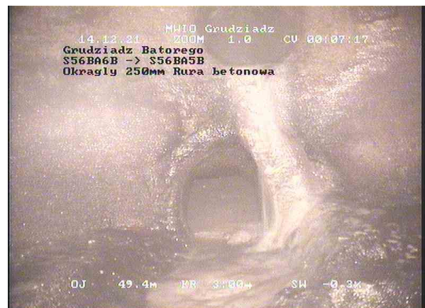
4c3aaa1b-3516-463d-a594-2508ea4f940b_20211214_154414_795.jpg, 00:05:58, 49.46 Studzienka wiazowa
