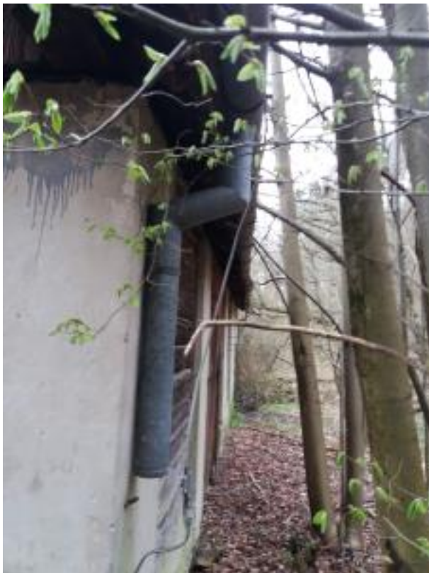
Oberwane rynny i rury spustowe
