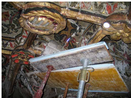
Protective and isolating layer between the wall painting and shoring in the church of Freixo de Espada à Cinta, Portugal, 2007. Photo: Esmeralda Paupério.
