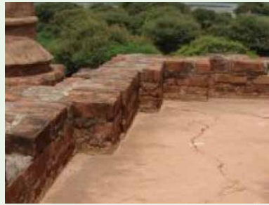
Cracks in the roof of a temple, Bagan, Myanmar, 2016. Photo: Eugénie Crété.
